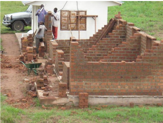
Dormitories, First Phase, in construction (Nov. 2009).
