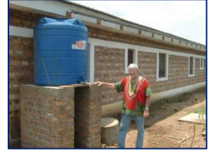
Fred Suter with completed eaves-trough system at Tshikapa Welcome Center
