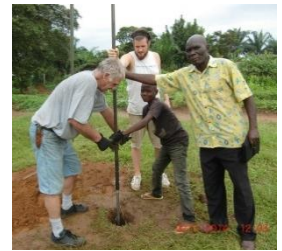
Les Schlegel, Daniel Suter, Dominique Yona and a young Congolese boy work at digging a small bore well
